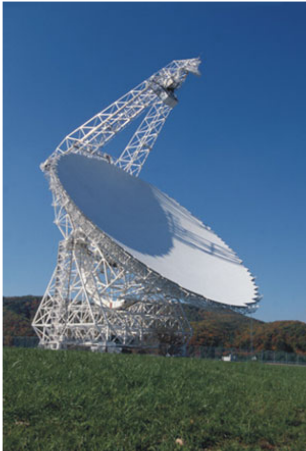
Green Bank 100m Antenna
